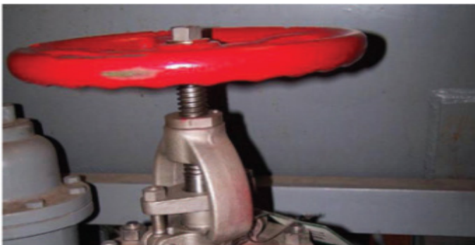
Counterfeit valve on the left with the red steering wheel. Legitimate valve on the right with the gray steering wheel. The differences are obvious to a discerning eye, but can escape an unsuspecting inspector.
